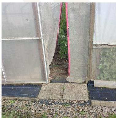
Typical Polytunnel entry
